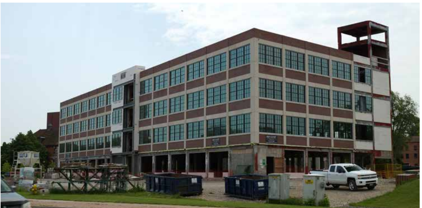
Image 2F: The adaptive reuse of the existing Walkerville Power Building is an example of sustainable development Image source: BrookMcIlroy
